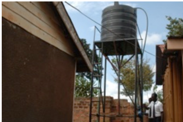
The cistern sits higher than the bathrooms, so the force of gravity moves water from the cistern to the sinks and toilets when needed.
