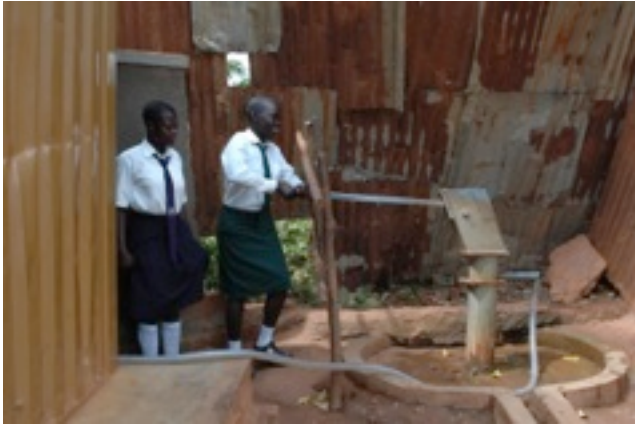
Students pump water from the well Mtaala installed in 2009. The water travels from the well through a hose to the manual pump.
